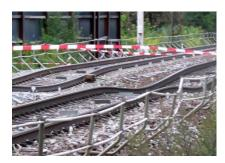
Earlier this week the already grim situation got suddenly worse, when tunnel construction in the town of Rastatt resulted in unexpected damage to the double track Rhine Valley mainline. The tunnel boring machine that was crossing a few metres below the railway line caused a serious deformation of the tracks, making them unsuited for traffic.
