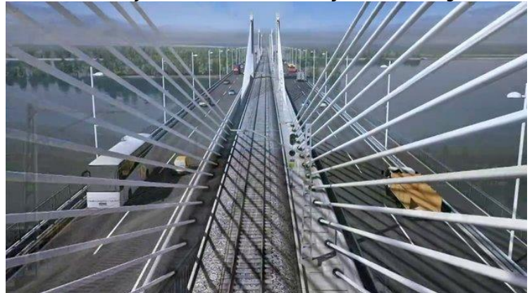
Railway line on the new Vidin-Calafat Danube Bridge
