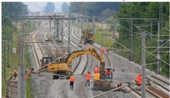
And then, on 12 August, disaster struck when the central section of the Rhine Alpine Rail Freight Corridor became unusable due to a man-made error near the town of Rastatt in Germany. Tunneling works under the mainline caused the rails above them, which handle up to 200 freight trains running between the ports of Rotterdam, Antwerp and Hamburg and Northern Italy, to severely deform.
